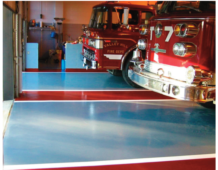
Firehouse floors have a Stonhard epoxy system with a urethane coating that is safe, improves cleanability, stain resistance and UV resistance while providing a glossy, sleek finish.
